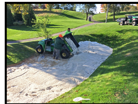
Making repairs on the bunkers
