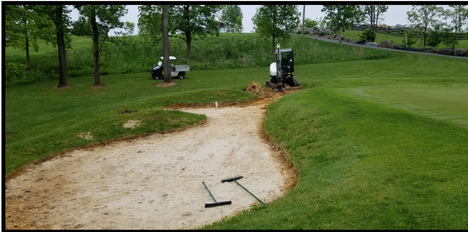
Above: Boulder No. 9 Bunker Repairs
