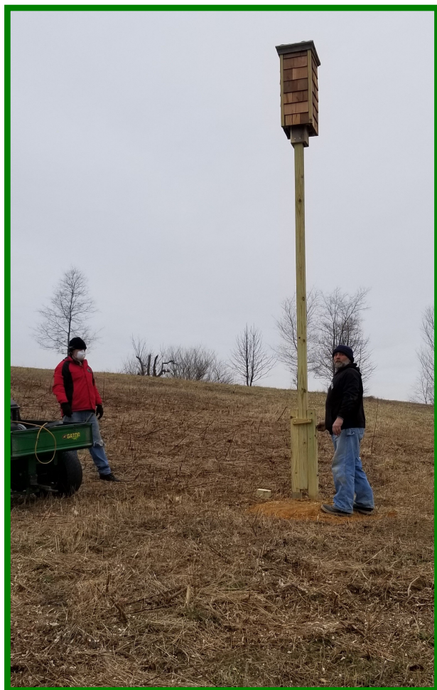
Installing the Bat Houses
