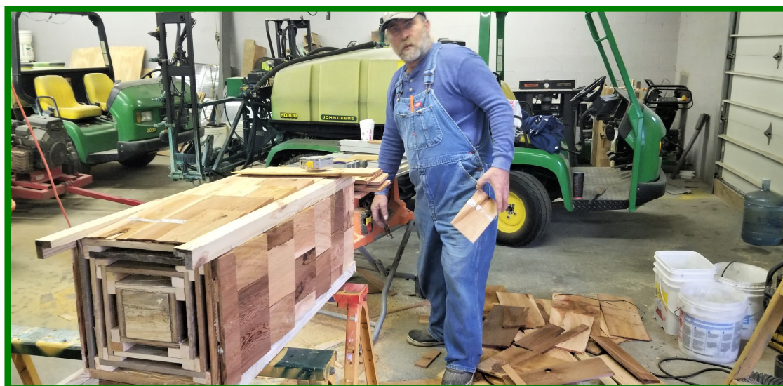
Constructing the Bat Houses
