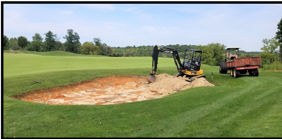
(Picture: Boulder #14 bunker renovation, left)
