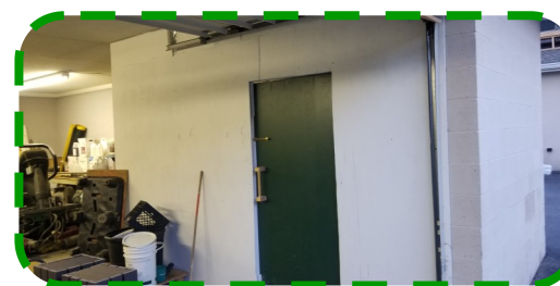
New chemical storage room, pictured above.
