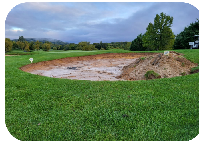
Starting Rock #11 Bunkers, pictured above.
