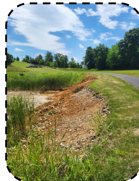
Rock 5 Pond Work
