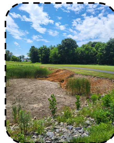
Rock 5 Pond Repair start
