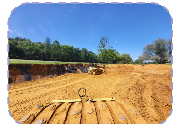
Rock 5 Pond Compacting Clay
